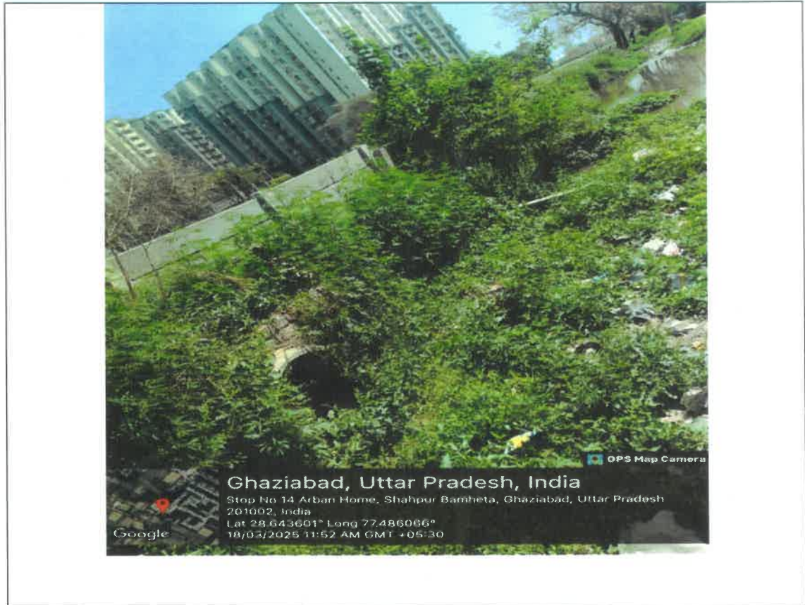
Pipeline near Group Housing Project Urban Homes
